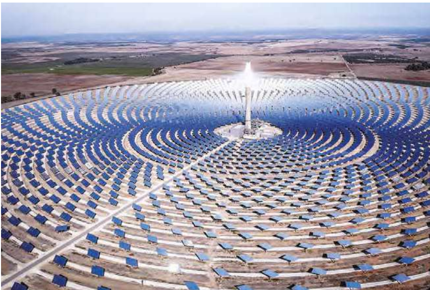
This solar plant in Fuentes de Andalucía, Spain, pictured on 17 October 2021, can supply uninterrupted power. Instead of sunlight, it uses solar heat (which is more easily stored) to generate electricity. SIMONE TRAMONTE
